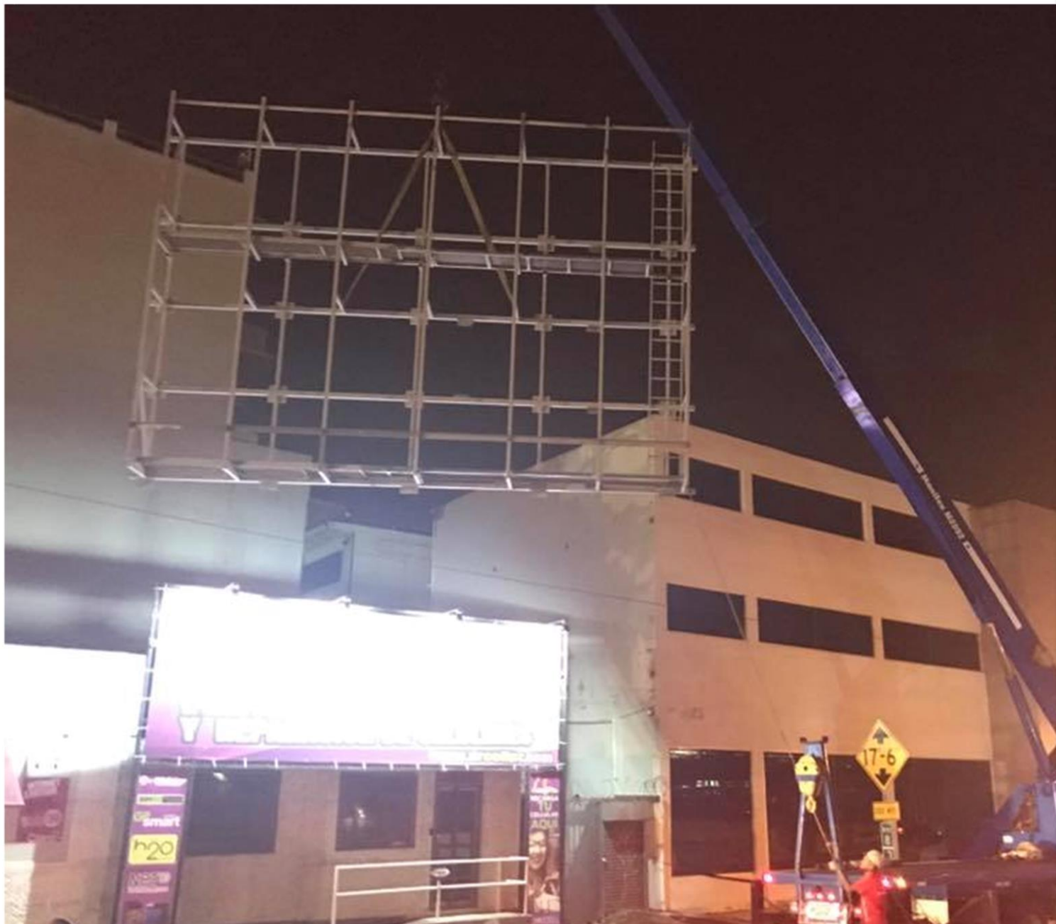
BILLBOARD STRUCTURE + DIGITAL DISPLAYS INSTALLATIONS @ HATO REY
